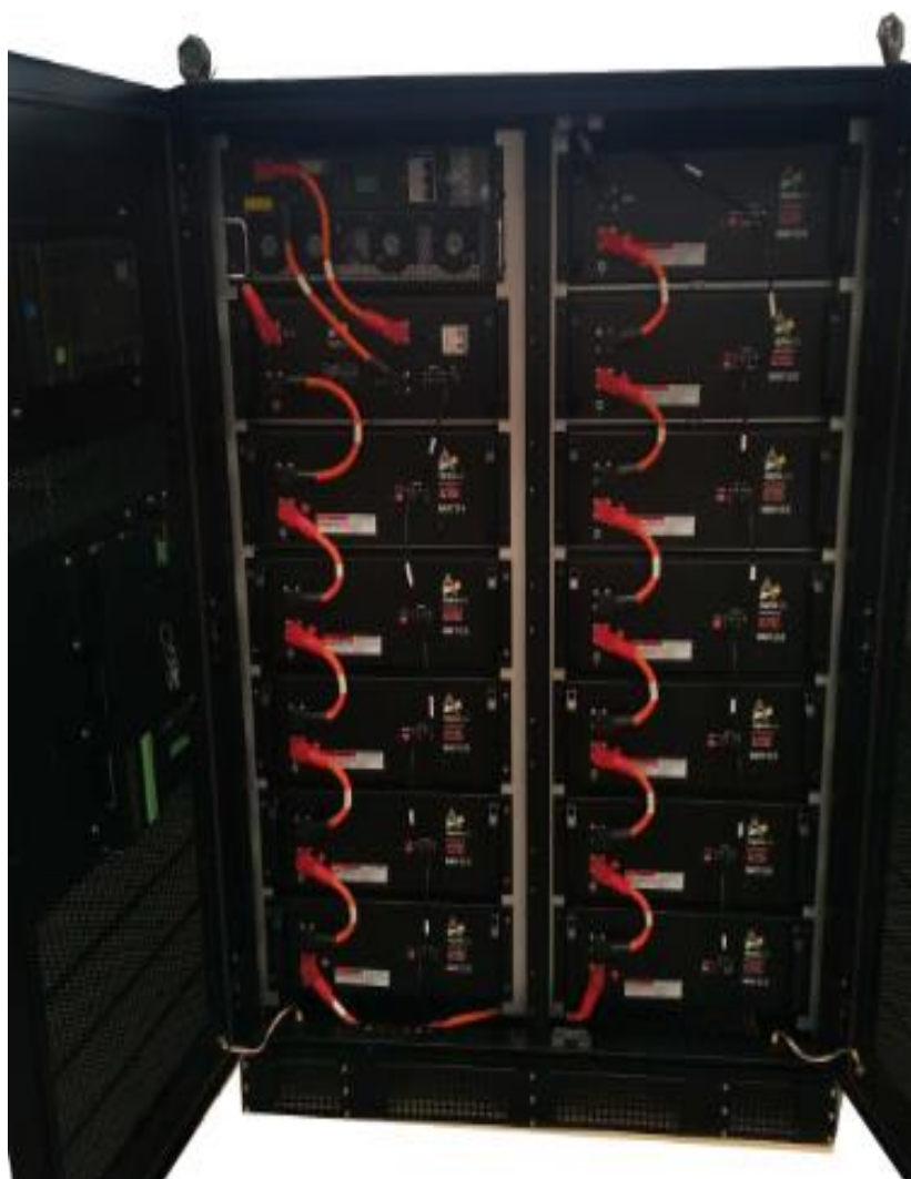
Figure 4.15 Completed installation of T30 System
